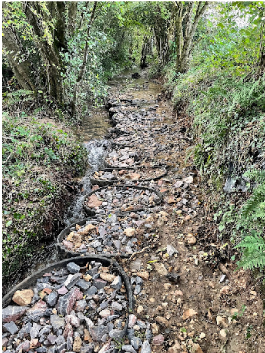
ADDITIONAL stone provides a sustainable surface whilst controlling stream flow
