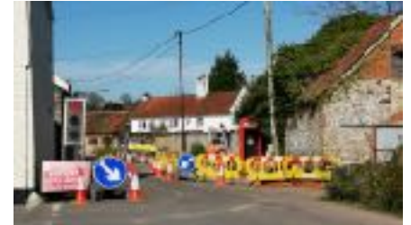
BROADBAND equipment being installed in Whitford
