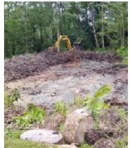
TURBARY pond clearance and Andy Podbery's new pond construction
